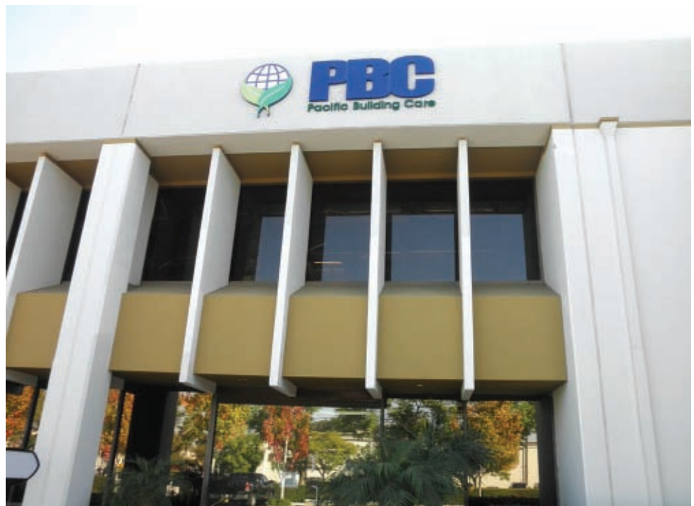
PBC assists professionals in achieving cost savings through energy efficiency
