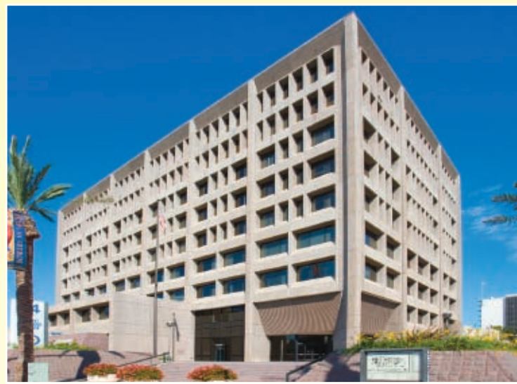
The Santa Ana Federal Building Local TOBY Winner Renovated Building Category
