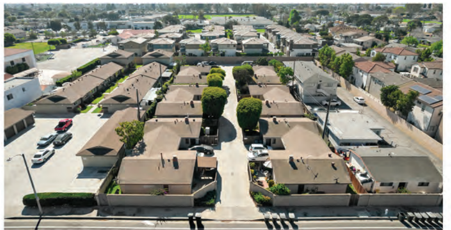
673 & 675 VICTORIA STREET | 12 UNITS | IN ESCROW Costa Mesa | $6,500,000
